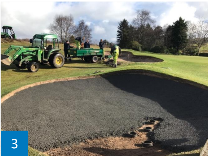
3 Spread Capillary Concrete® at 2-inches
